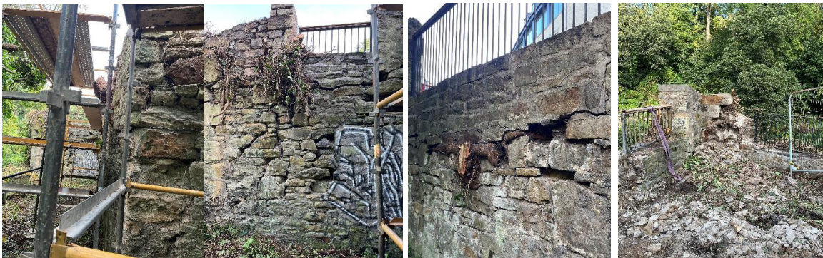
Miller Row Clearance and Issues (during)
